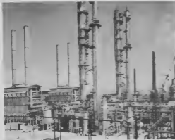
Hydrogen Plant No. 1 (in foreground), located north of Powerhouse No. 1, is ready to go on stream in March. Next to it is Hydrogen Plant No. 2 which is scheduled for startup in April.
